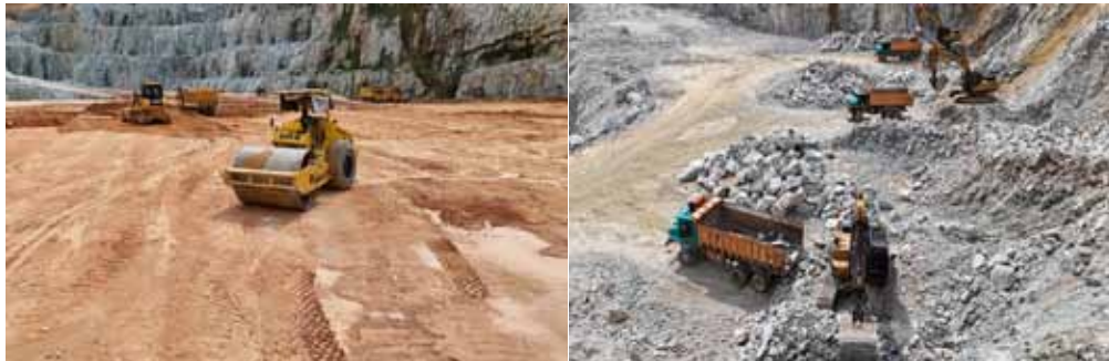
Cut and fill, and compaction
