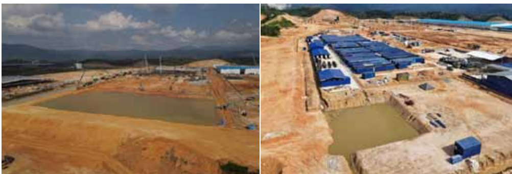
Erosion and sediment control plan
